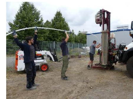
Construction of monitoring and sample sites (MET department, UFZ)
